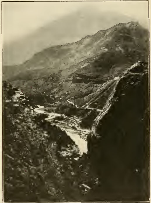
General View of Maitenes Generating Station Under Construction Showing Steel Penstocks
